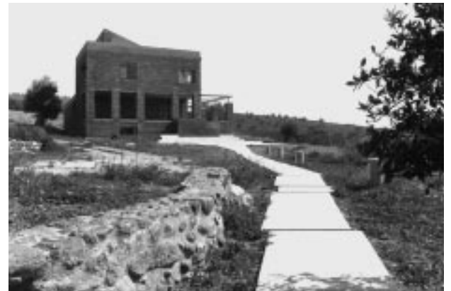
Mavrakakis Art Studio: Main access to the building
